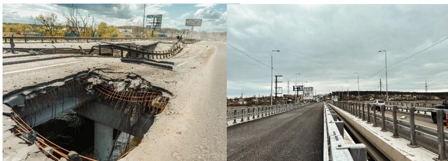
Fig. 1: Gostomel bridge in 2022 and 2024. Photo - Ministry of Infrastructure
