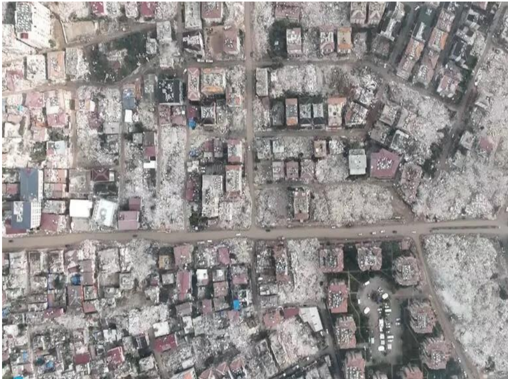
Figure 1: The Degree of Damage of the Old City of Hatay
