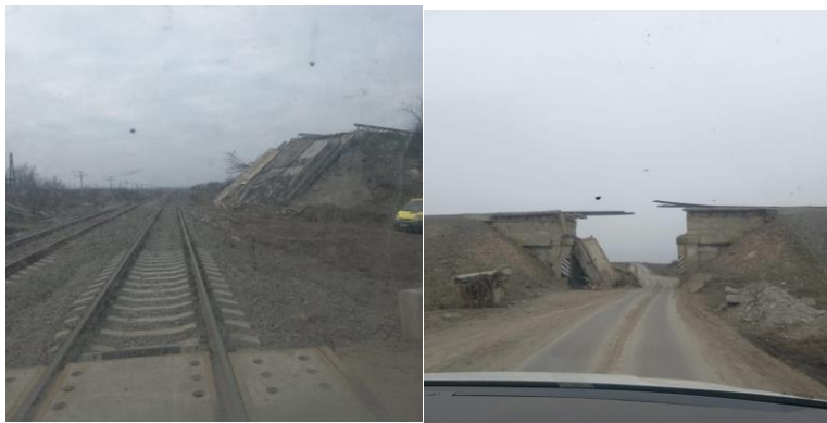
Fig. 3: State of bridge structures on the front line
