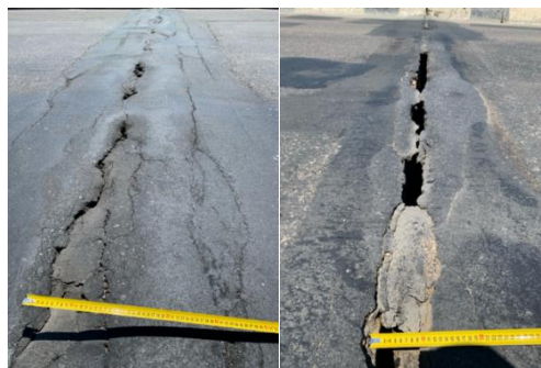
Fig. 12: The state of the deformation seam
